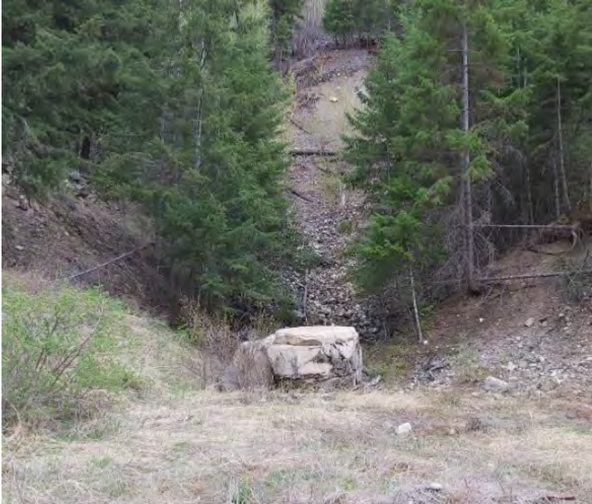
Figure 10. Site of Copper Farm Adit #1, now collapsed
